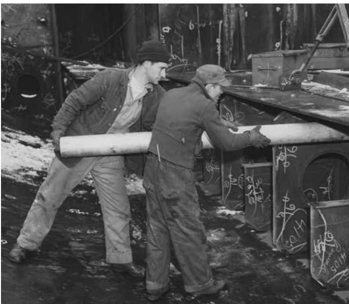
Shipyard workers building an aircraft carrier, Newport News Virginia, January 21, 1944. (Image: The National WWII Museum, 2011.102.411.)
