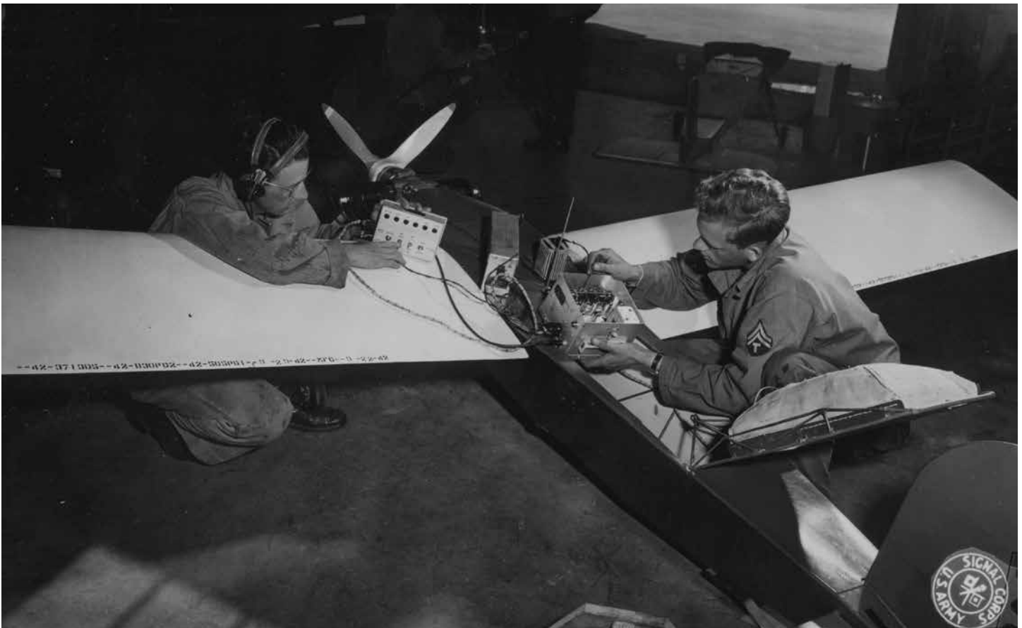
Soldiers making adjustments to a radio transmitter and receiver on a radio-controlled target plane. (Image: The National WWII Museum, 2011.065.1176.)
